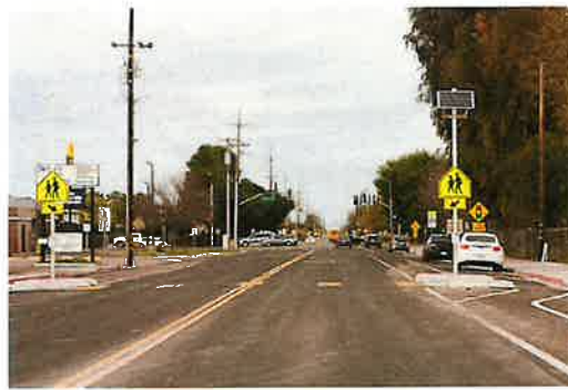
RRFBs on Dairy Avenue in Corcoran
